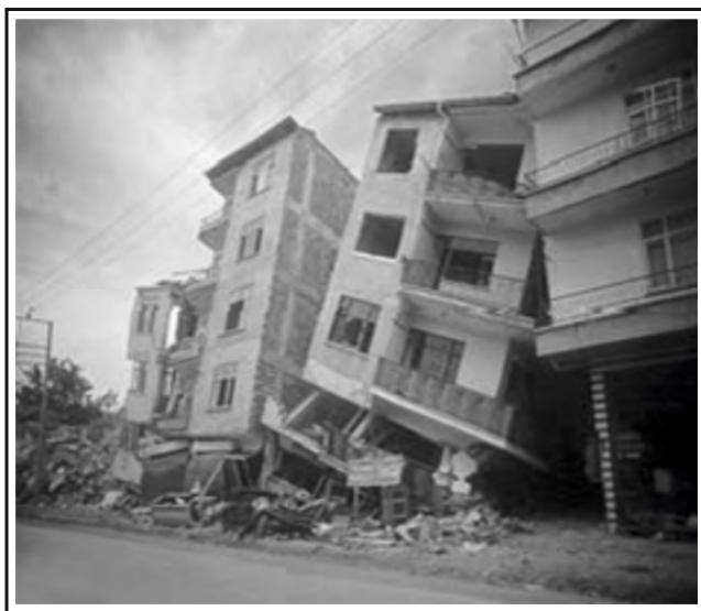
Fig. 3. Failure - Stilt Floor
