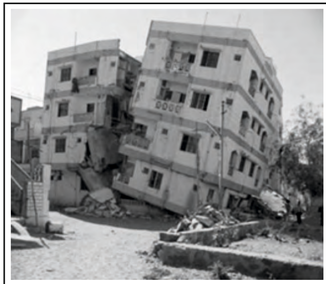
Fig. 4. Failure - Soft Ground Floor
