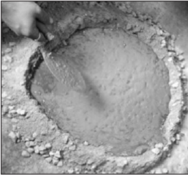
Fig. 9. Wet Mixing
